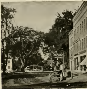
MAIN STREET LOOKING TOWARD BRIDGE
